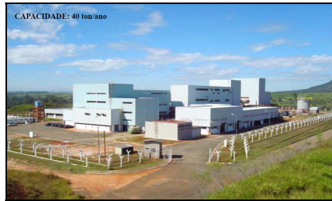
Demonstration Conversion plant USEXA/CTMSP
